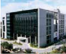
Taoyuan Technology Center (Green Building)
